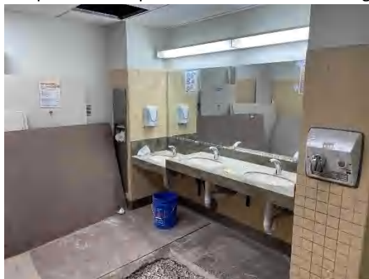
Men’s Restroom Existing Finishes
