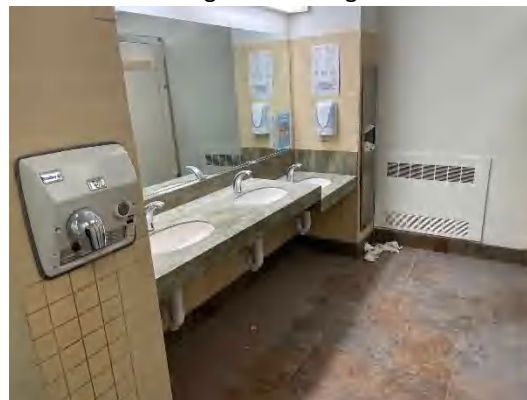
Women’s Restroom Existing Finishes
