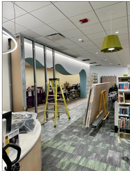
Temporary wall coming down
